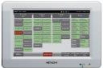
Central Station EZ
